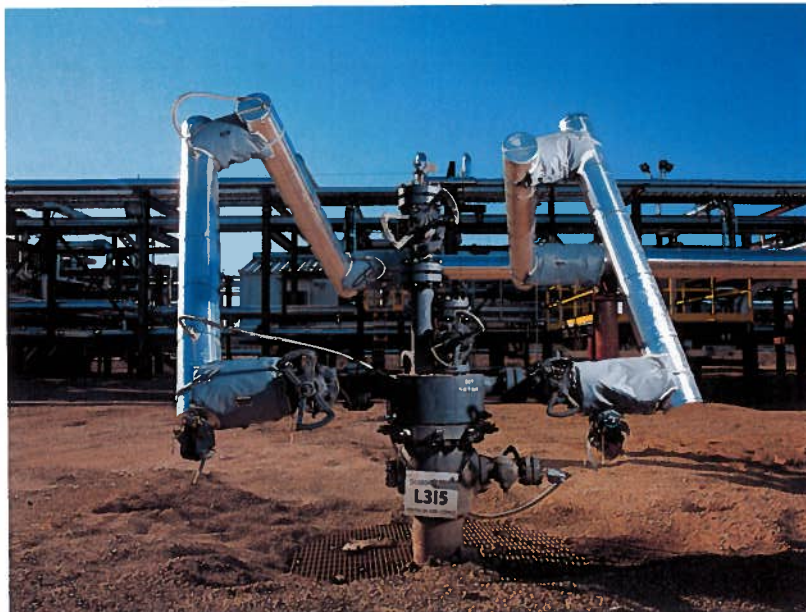
Statoil, led by Canadian operations chief Lars Christian Bacher , is blasting steam into wells, like the one above, to dislodge Alberta's bitumen from sand below ground.
